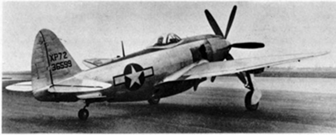
XP-72 No.2 (43-6599) with six-bladed contra-rotating coaxial propeller.
